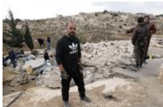
Jabbar Dababsi in front of his demolished home this week. Credit: Alex Levac
